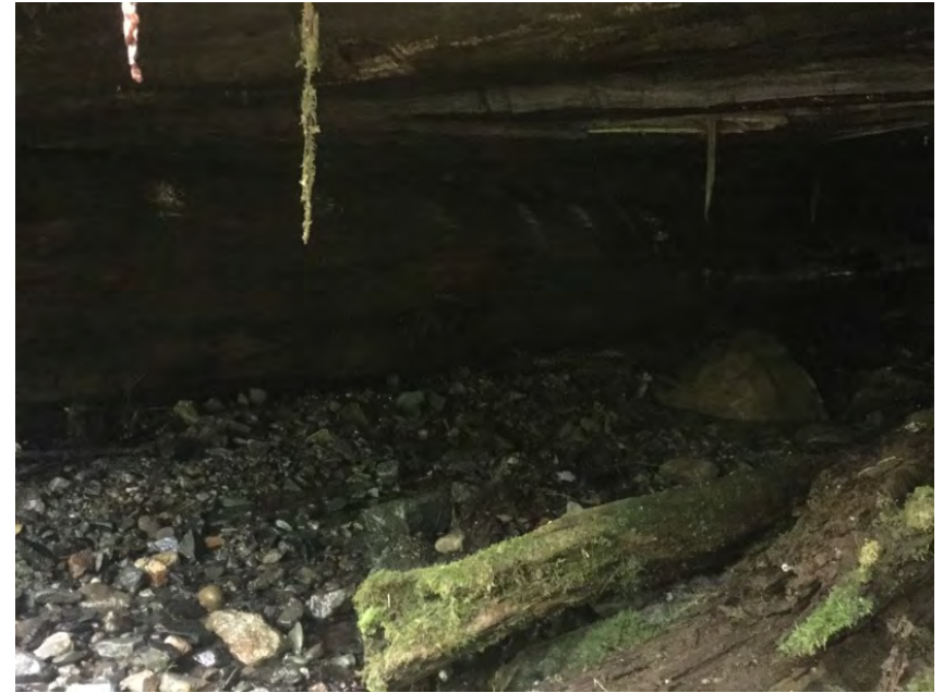
Right Bank Abutment when facing downstream
